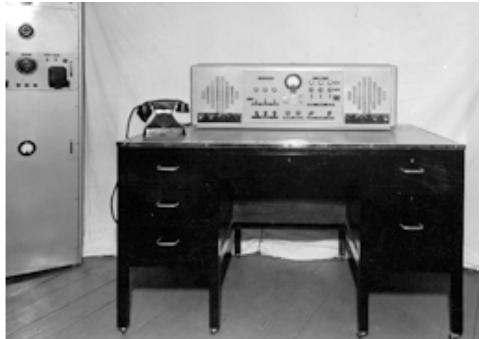
Lancon-built HQ Control panel. pre 1957
